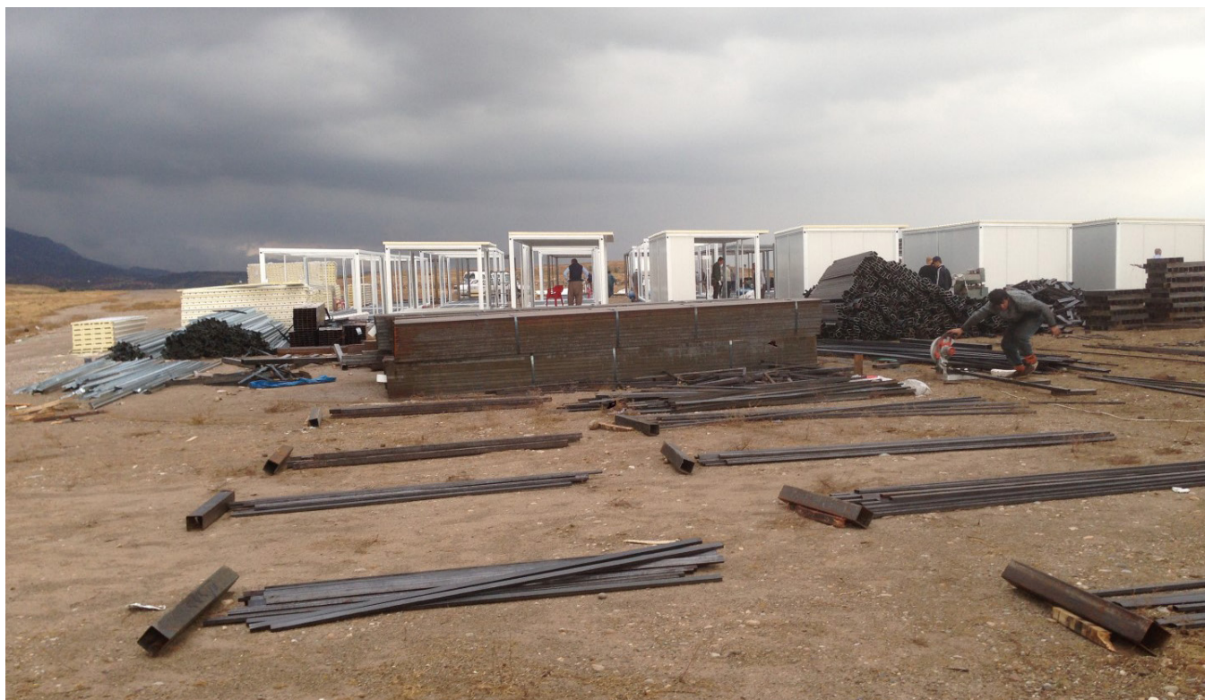
Shelter units construction in Barzanja Camp in Sulaimaniya
